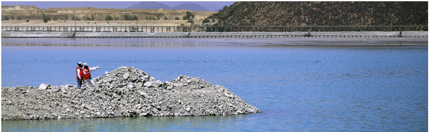
The El Torito tailings facility at El Soldado, Chile.
